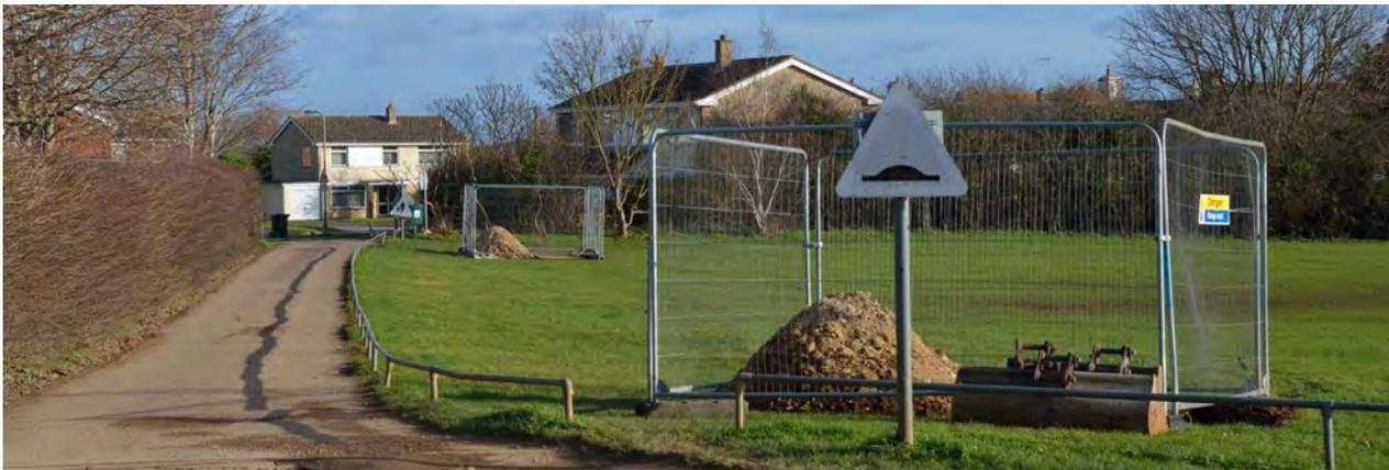
You may have seen some temporary excavations in the field in mid-January (above); test holes were dug to establish ground conditions ahead of construction, and they were refilled when the survey was completed.
