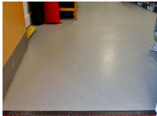
We have also had the store area re-floored (above right) as we had been facing problems due to wear of the floor paint and erosion of the concrete underneath. The new flooring is a commercial-grade durable PVC material, which should give us an extended period of service. It is looking good.
